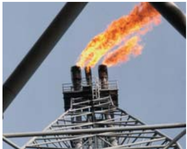
Today's refineries and chemical plants frequently burn-off waste gases in a flare line. Because both flow rates and gas compositions vary, the TA2 can be used to obtain relative flow indication.
